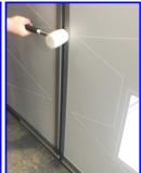
Assemble the central shower cubicle first – start with a door panel, and slot into the grooves of two adjacent base trays; now slot a corner post into place, and slide a wall panel against the door panel and base. Continue until the cubicle has all its door and wall panels secure.
